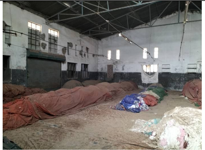
Internal View of Factory Shed.
