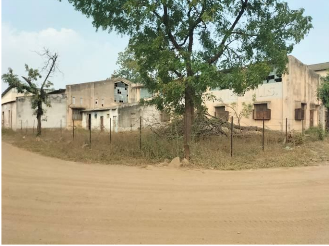
External View of Industrial Factory Shed.
