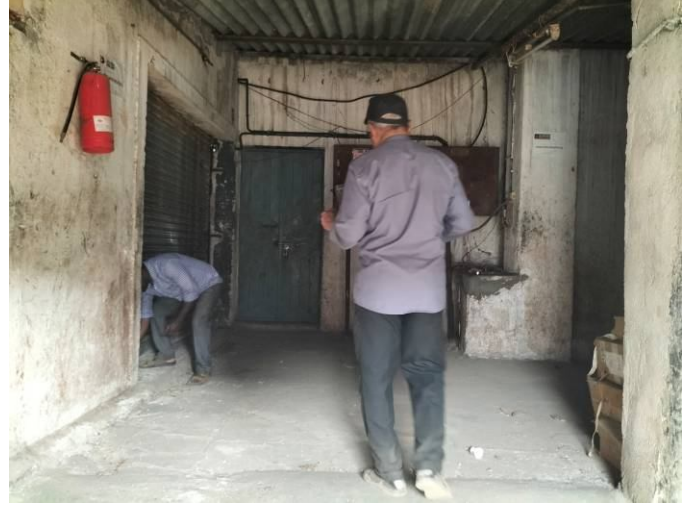
Internal View of Industrial Shed.
